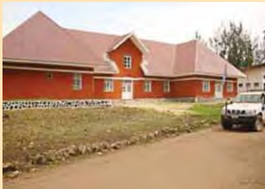
Local administration building constructed with support from MONUSCO in DRC
